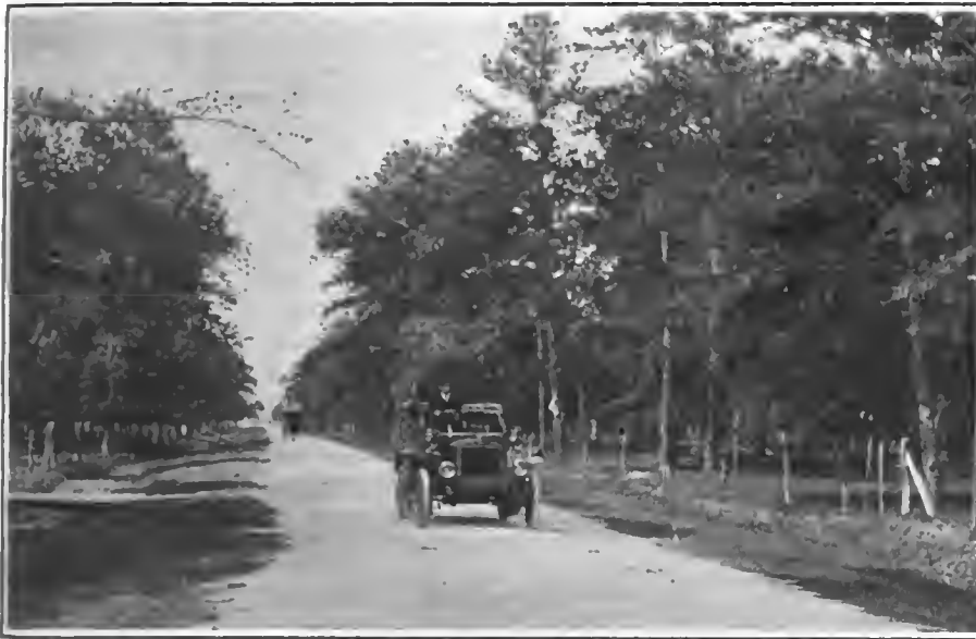
DRIVING ON THE SHELL ROAD NEAR HOUSTON, TEXAS.
